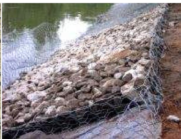
**Fig. 10.** Use of Reno mattresses for scour protection of embankments
