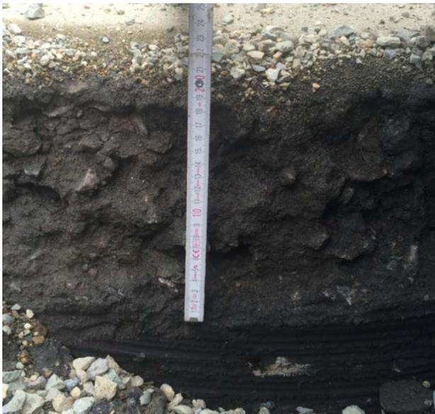
**Fig.** Transverse cut of a road structure
