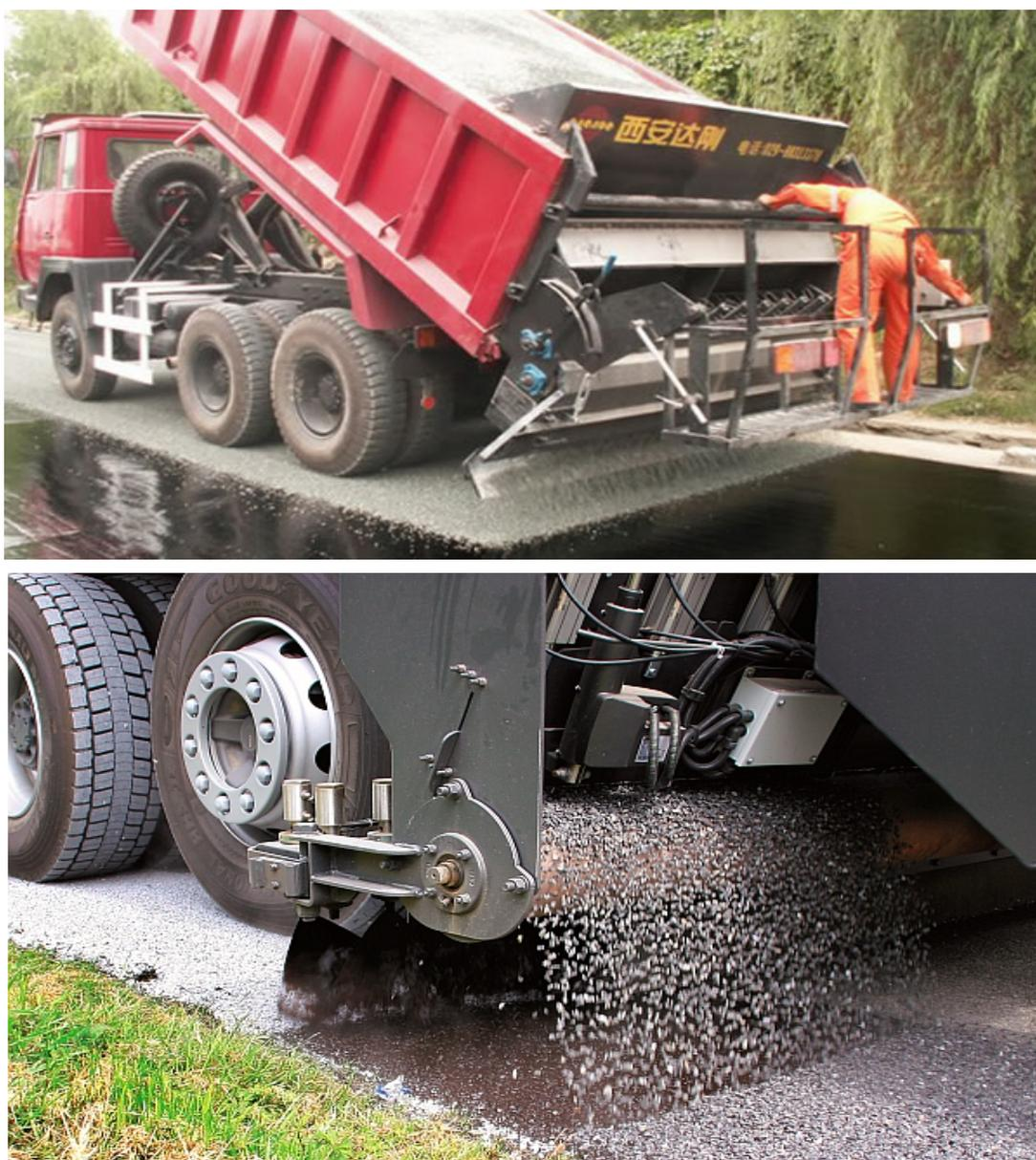
**Fig. 1.** Options for the backward and forward operation of bitumen crushed stone distributors
