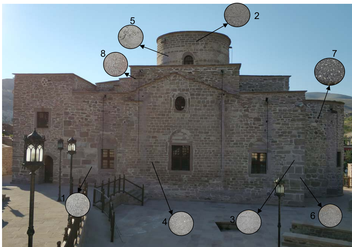
Fig. 2. South-West Side of the Aya Helena Church and Petrographically Different Building Stones
