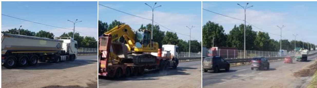
Fig. 3. Transport flow in the surfacing repairs site
