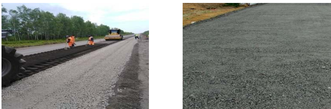
Fig. 4. Construction of road pavements using asphalt-granular concrete mixtures in the Tambov region (photo by the authors)
