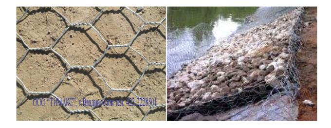
Fig. 9. Mesh of double twisting with hexagonal grids for Reno mattresses, Ltd. Timaks, Vladivostok **Fig. 10.** Use of Reno mattresses for scour protection of embankments
