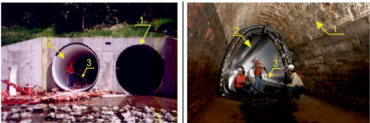
Fig. 5. Examples of structures made designed SPR SL technology: 1 — body of the drainage pipe (collector) before reconstruction; 2 — collector body after the application of the wound technology; 3 — typical element of SPR SL technology
